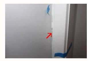
Poor finish to internal corner at both sides of wall adjacent to wardrobe frame.
